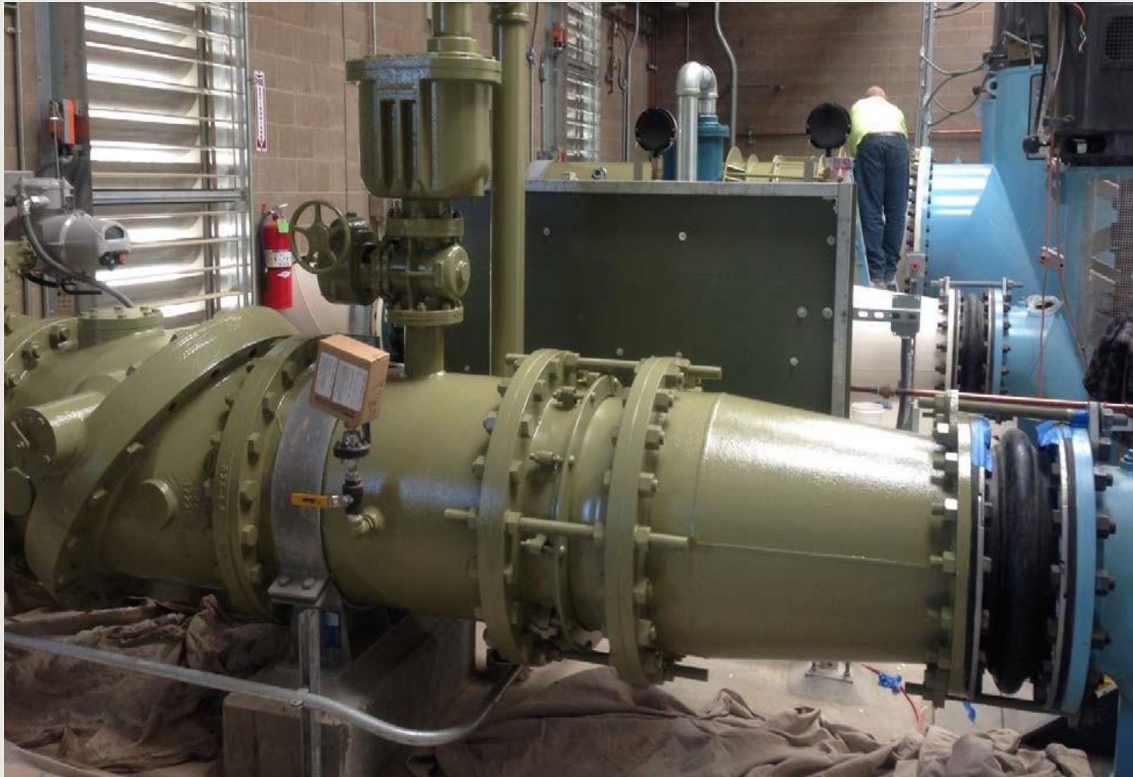
Joint Intake Raw Water Piping in Pump Room
